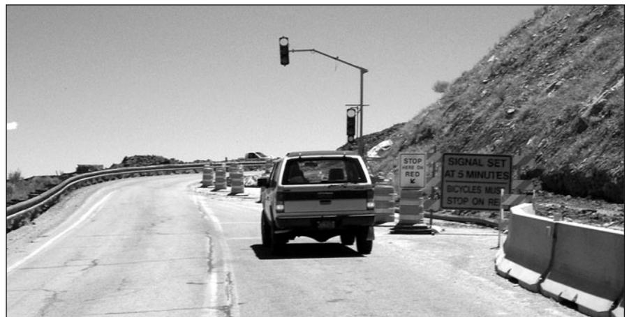
Figure 6. A portable traffic control signal providing one-lane, two-way traffic flow around a construction zone.
